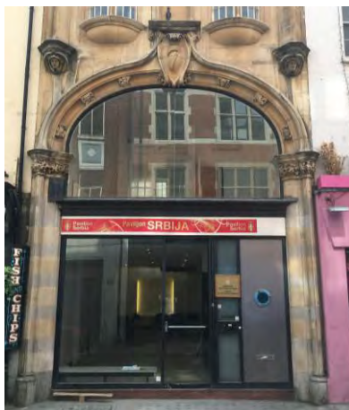
Picture 2. Existing stepped entrance
