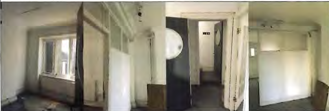
PHOTOS OF EXISTING STATE
