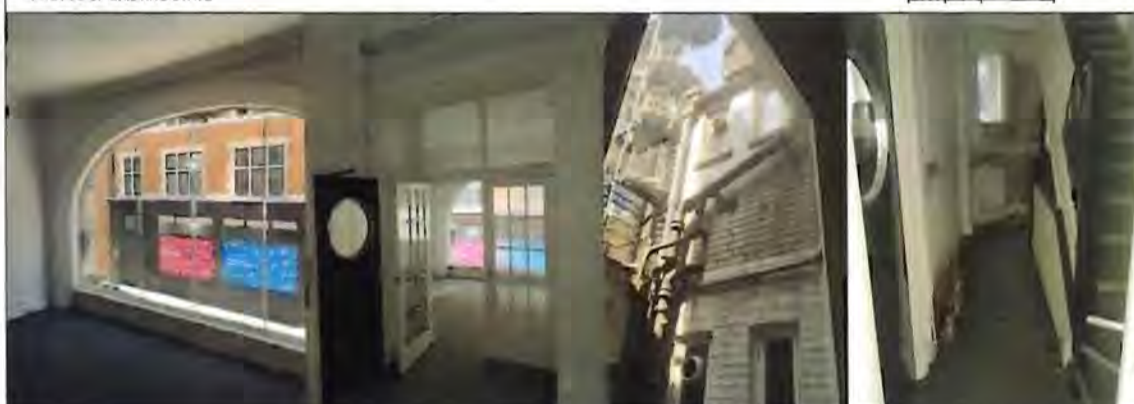
PHOTOS OF EXISTING STATE
