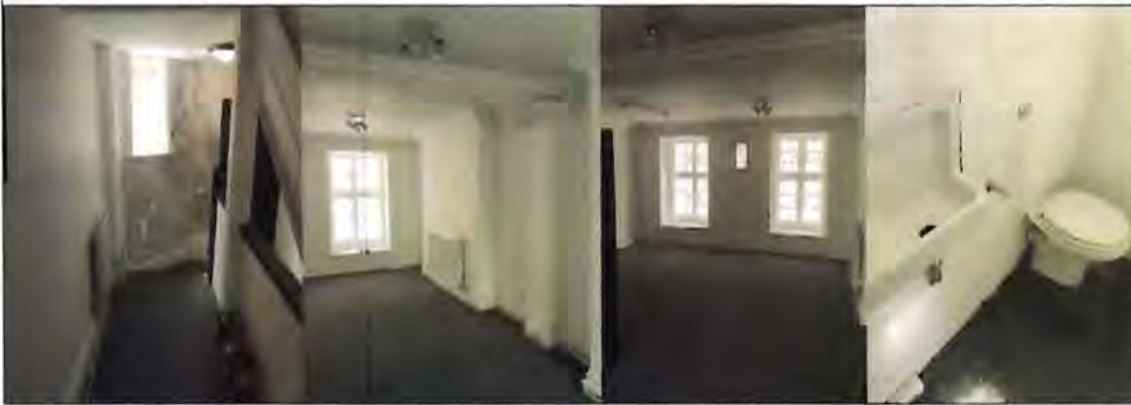
PHOTOS OF EXISTING STATE
